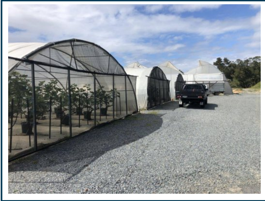
Photograph 3 – Looking south across greenhouses.
